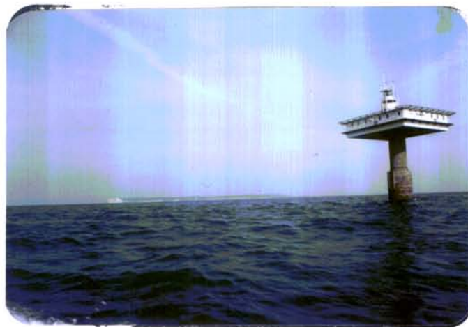
Photo 1: The Royal Sovereign Light Tower with Beachy Head in the background.
